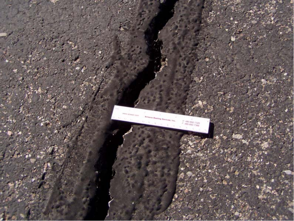
Runway 30R Safety Shoulder (west side), using 6" ruler
